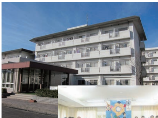
▲International House Building A
